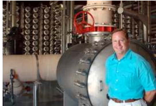
Christy Espinosa/Valley Morning Star Bill Norris of NRS Consulting Engineers in Harlingen has been instrumental in developing plants that turn brackish water into drinking water. His next project is to build a desalination plant on South Padre Island.
