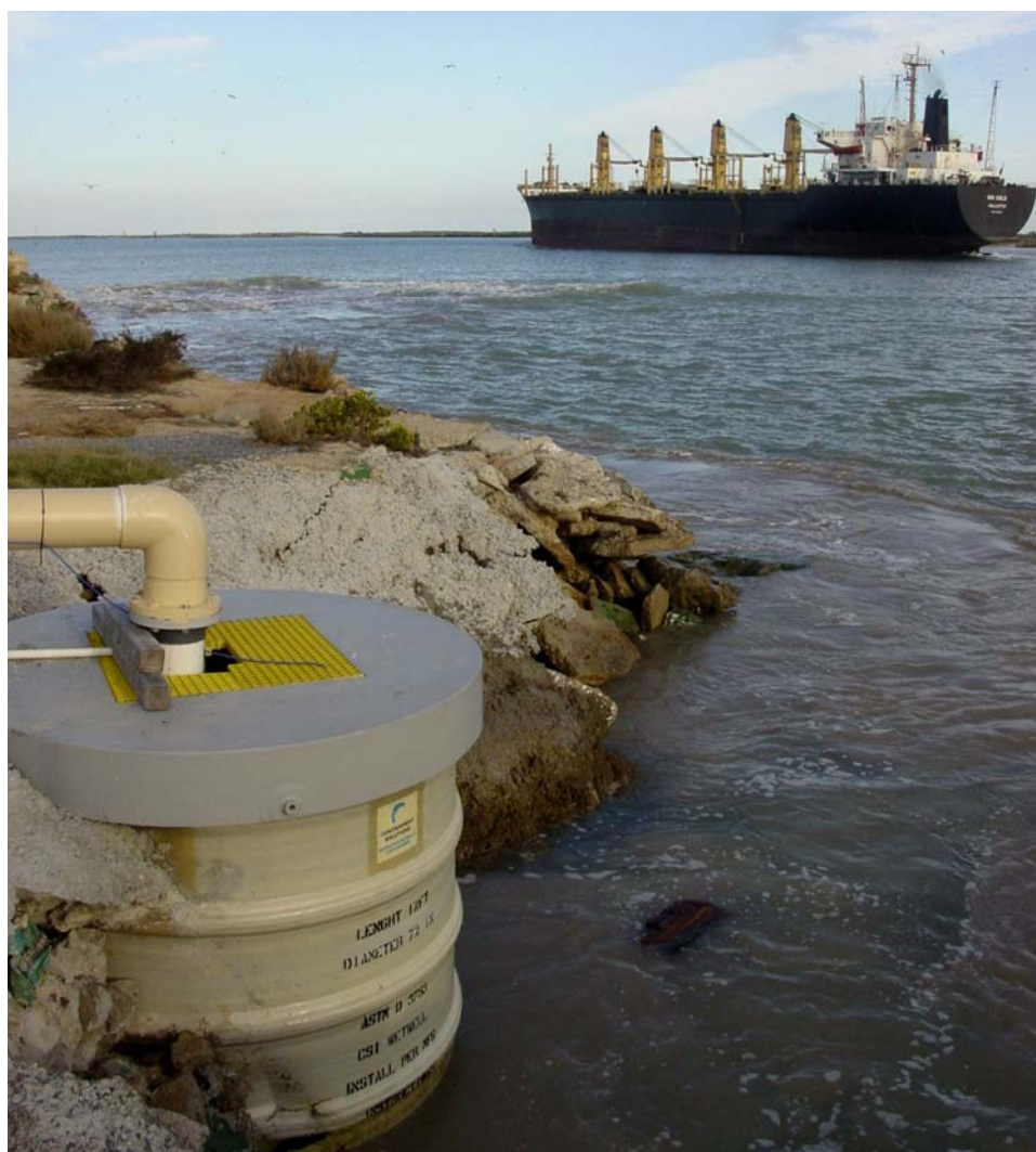
Figure ES-3: Photograph of the effect of a cargo ship passing on raw water turbidity in the Brownsville Ship Channel.
